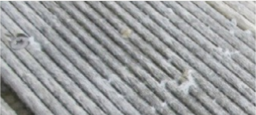
Natural occurring surface fibres on decking
