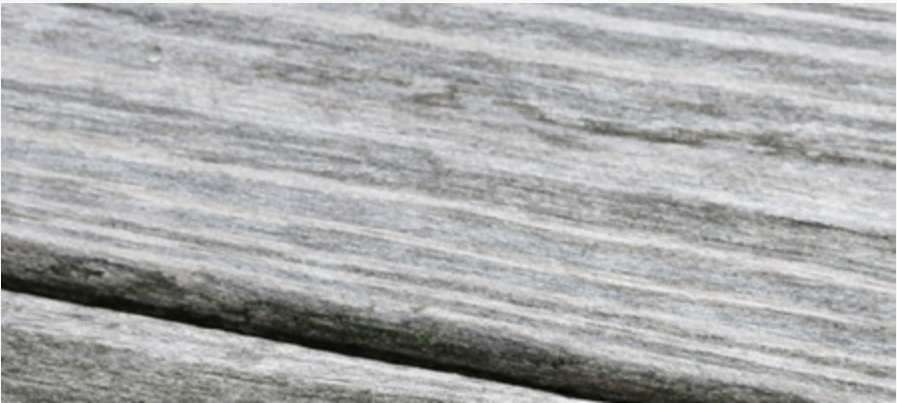
Natural occurring surface fibres on decking
